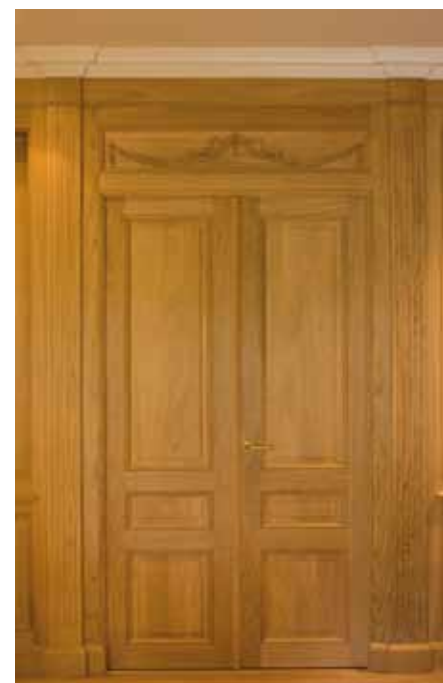
A double door integrated into the panelling with a hand cut oak garland above it.
